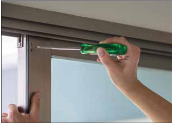
Easily adjustable outer-panel lock
