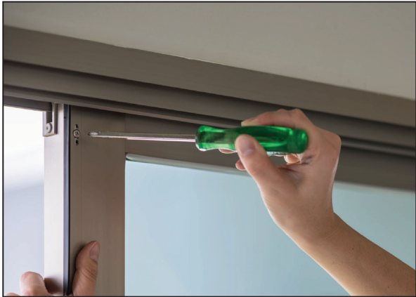
Easily adjustable outer-panel lock
